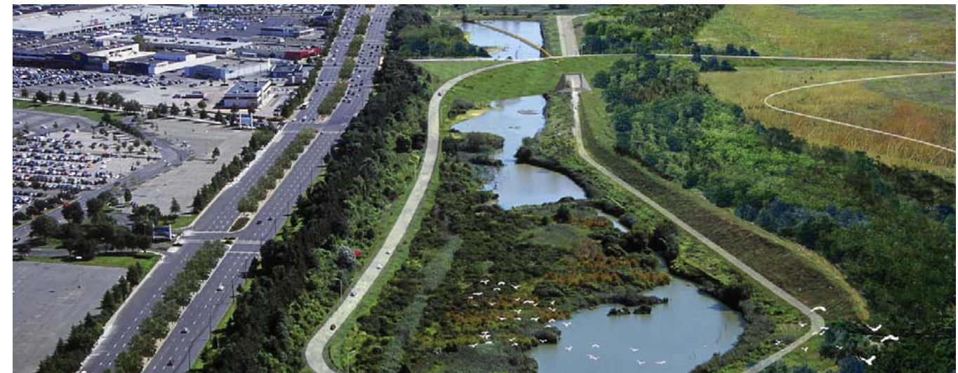
FIGURE 23: ILLUSTRATIVE VIEW OF PARK DRIVE ALIGNMENT B LOOKING SOUTH ALONG RICHMOND AVENUE
