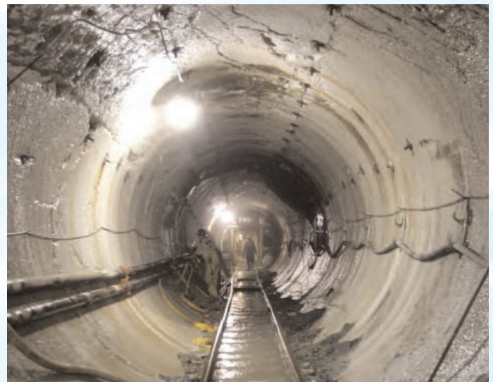
Tunnel No. 3, Manhattan, NY
