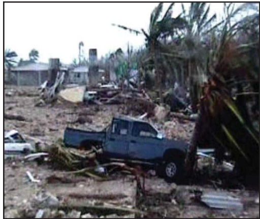
Figure 3. Total damages from Heta are estimated between U.S. $24 to 30 million, a total more than five times Niue's annual budget. (Source: SOPAC.)
