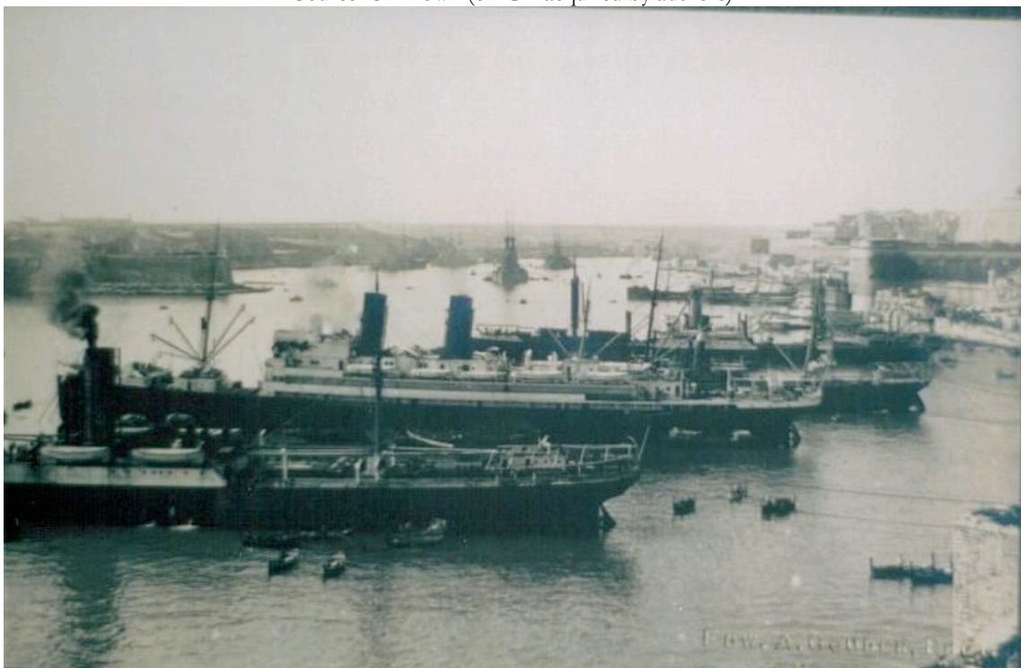
Figure 3. View of the Grand Harbour, Valletta ca 1900 Source: Unknown (on CD acquired by authors)
