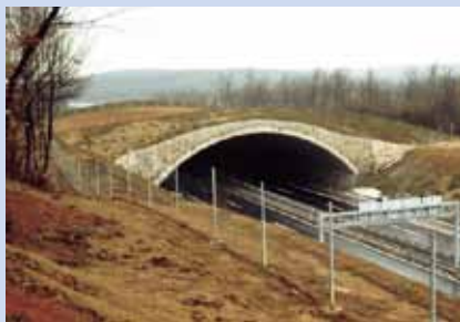
'Green bridge' over the highway enables animals to cross this barrier that crosscuts their habitat (photo: \. Huber)
