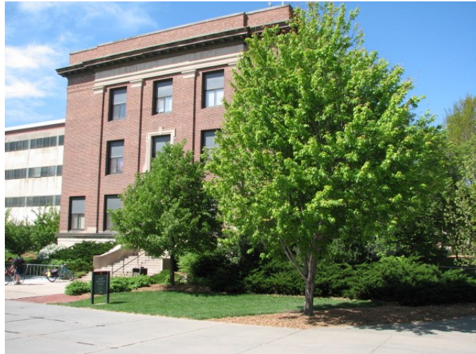
Canfield Administration Building Location of IRP
