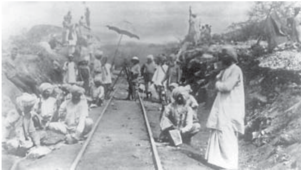
Indian workers surveying land after laying tracks, in Kenya. 31,983 workers went from India to Kenya between August 1896 to December 1901. 2,493 died in the construction, that is, four workers died for each mile of railway line laid; more than 38 dying every month during the entire six years. A further 6,454 workers became invalid
