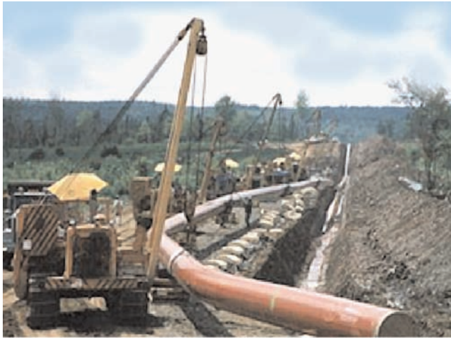
Figure 7 - Pipeline construction for transporting natural gas
