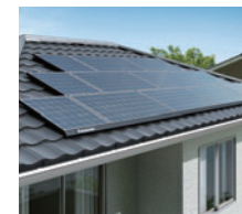
Solar photovoltaic systems
