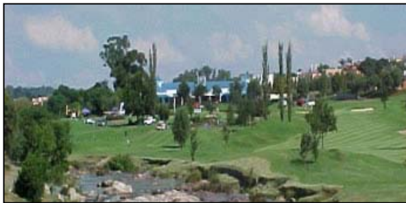
Figure 12: Golf course and clubhouse in Dainfern (Dainfern website)
