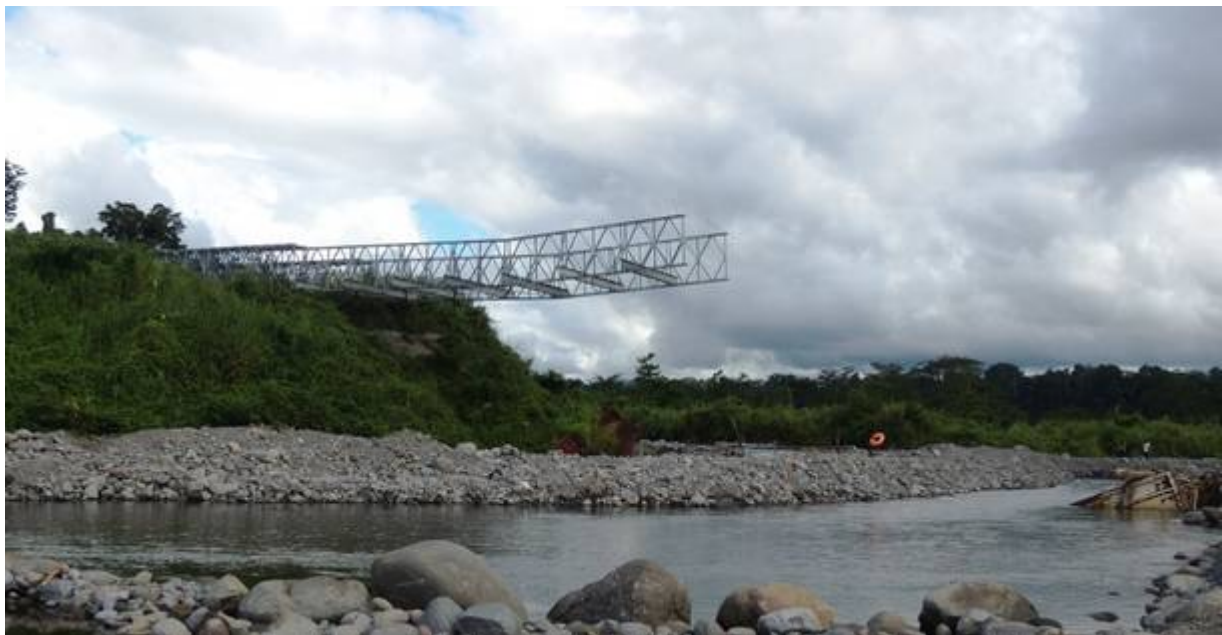
Part of Oro Province's long-unrestored main road and bridge infrastructure
