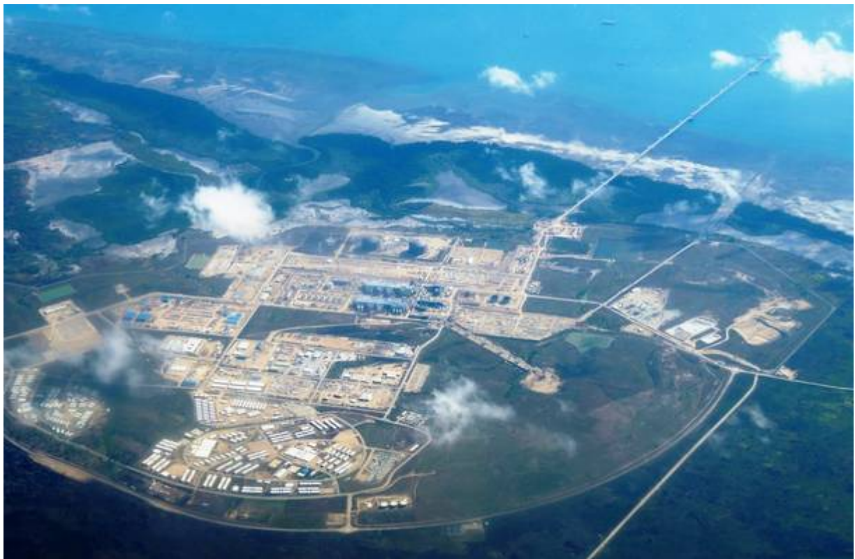
PNG LNG plant site and marine terminal under construction, in Central Province
