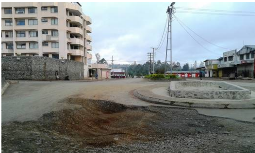
Potholes and trenches in PNG's rural and urban roads; here the centre of Mt Hagen city
