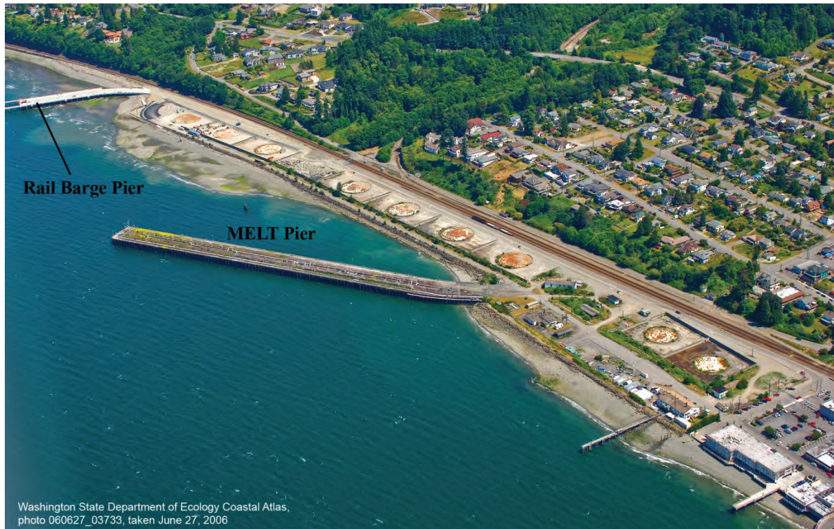
Figure 17. Overview of project area, 2006, showing Rail-Barge pier, pads from fuel tanks, and the MELT Pier.
