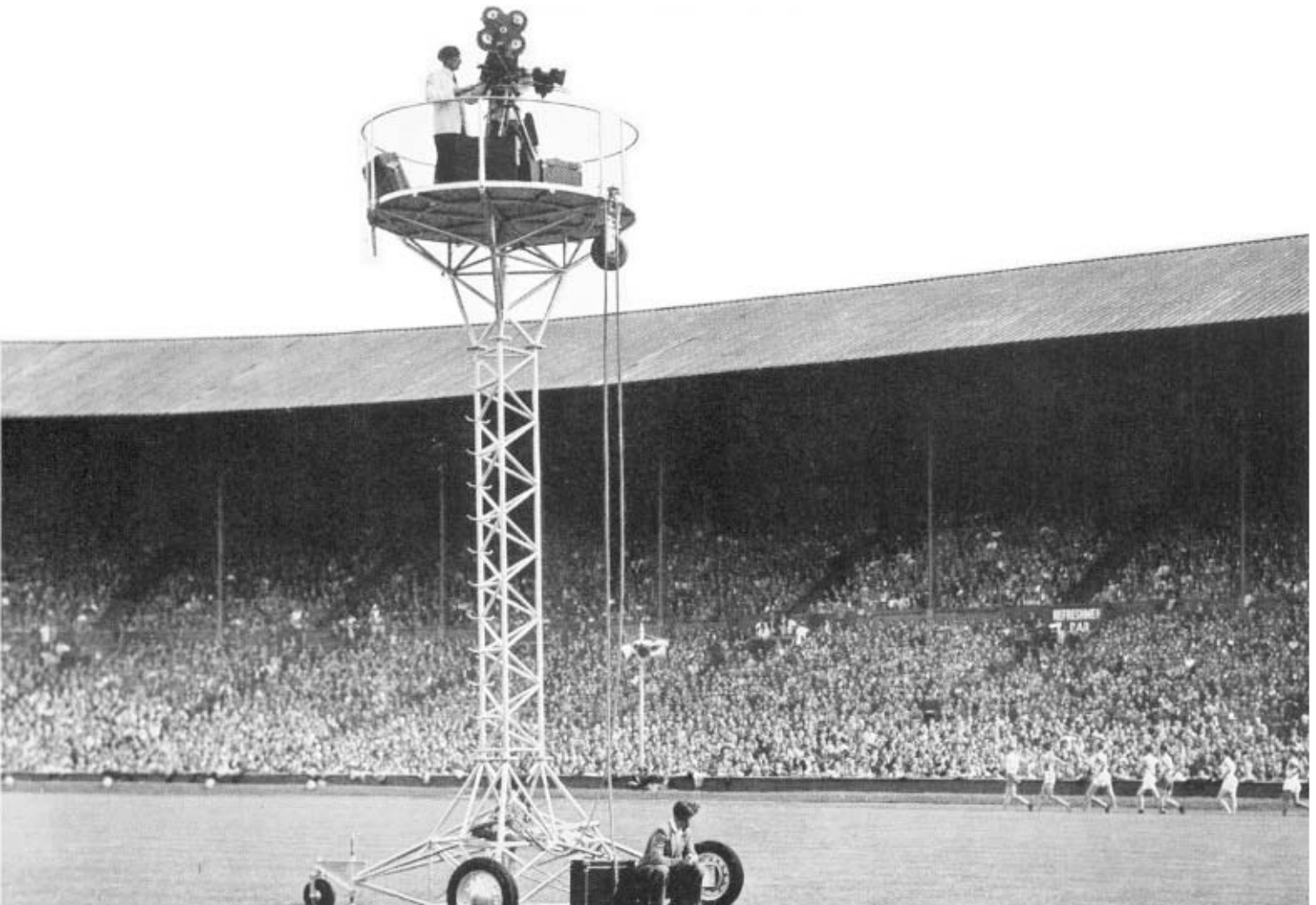
While the 10,000 metres walk is in progress, the film cameraman is busy on the top of the 24 foot portable tower which could be moved to the most effective vantage point for a particular event. The pulley apparatus at the side of the tower was used for hoisting camera equipment.
