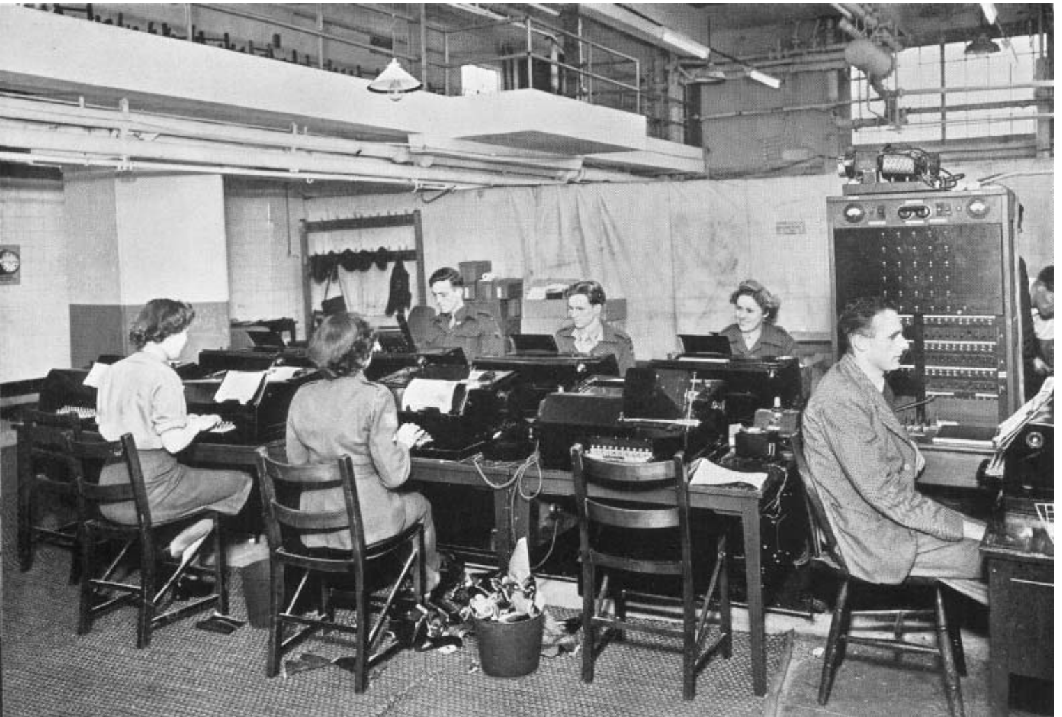
The teleprinter network at Wembley which enabled contact to be kept between the various Olympic offices, arenas and housing centres, and by which results and official instructions and messages were transmitted.
