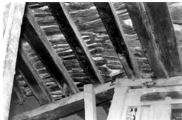
Fig. 97. Laths above the rafters.
