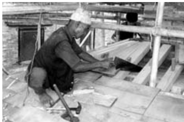
Fig. 98. Planking above the rafters.
