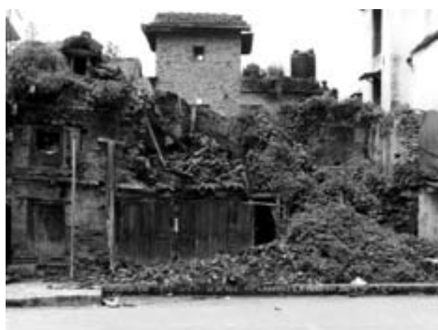
Fig. 41. Damage from water penetration.
