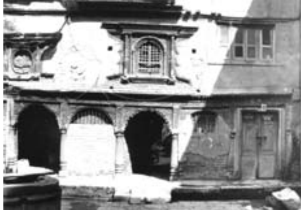
Fig. 62. Settlement of beam.
