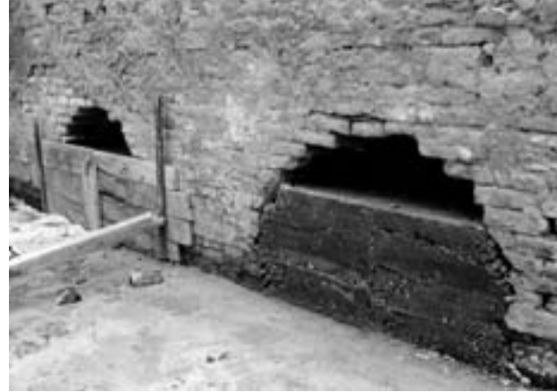
Fig. 88. Inserting damp proof course.
