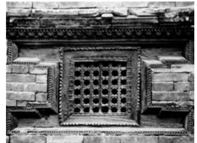
Fig. 72 Glazed shutter in lattice window.
