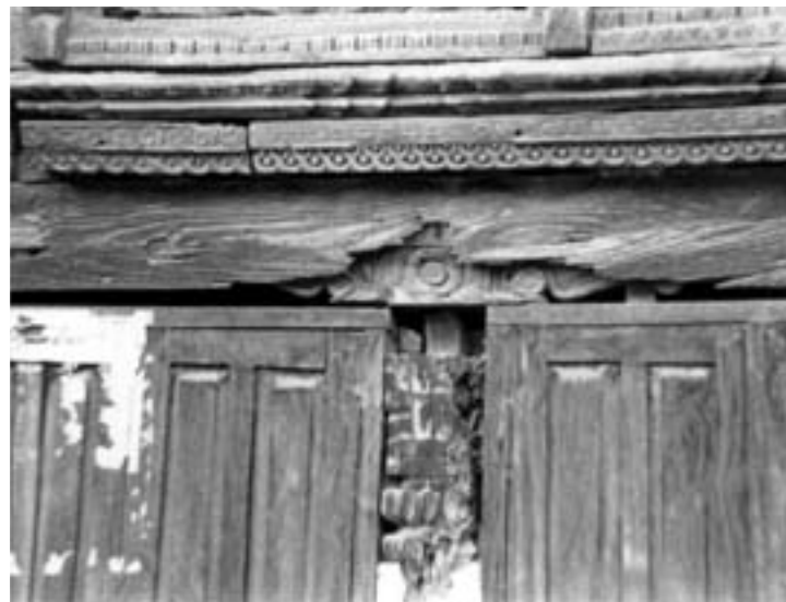
Fig. 44. Deterioration of timber elements from insects.
