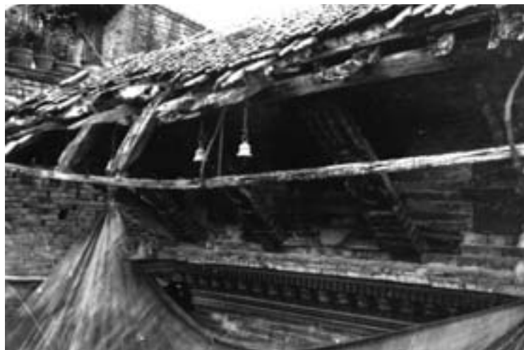
Fig. 51. Decay of eaves board.
