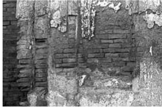
Fig. 100. Damage to plaster by ground damp.
