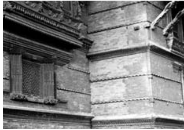
Fig. 92. Joints between new and old bricks.
