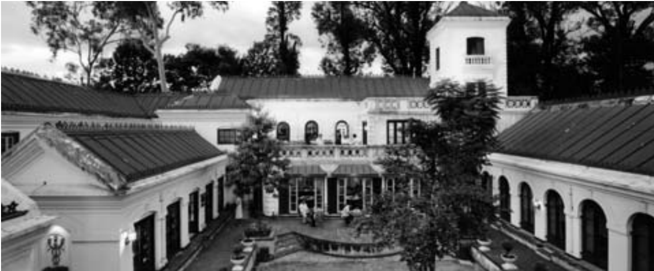
Fig. 25. Adaptive re-use for shopping complex.
