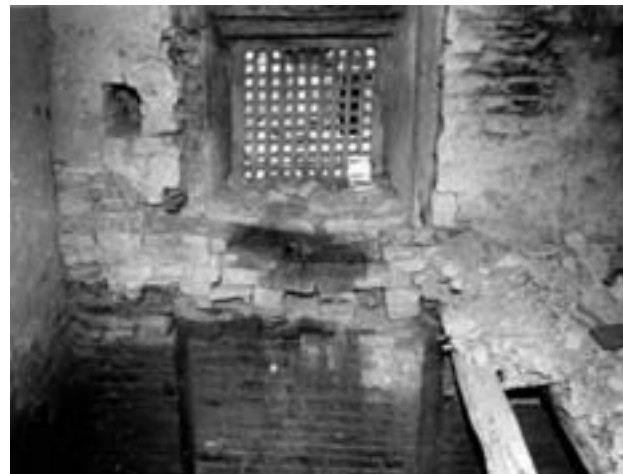
Fig. 49. Damage from ground damp.
