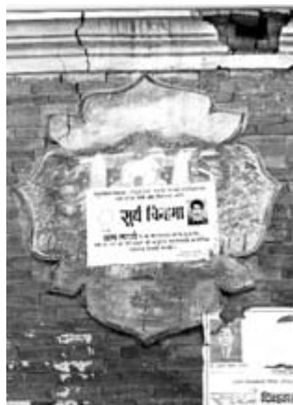
Fig. 4. Repair in situ saves historical fabric.
