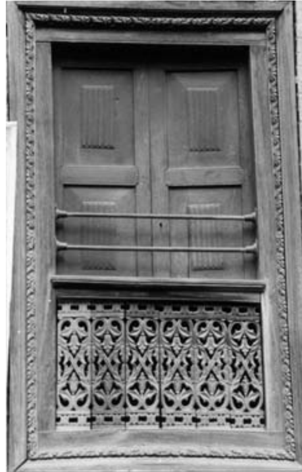
Fig. 70. Repair of carved elements.
