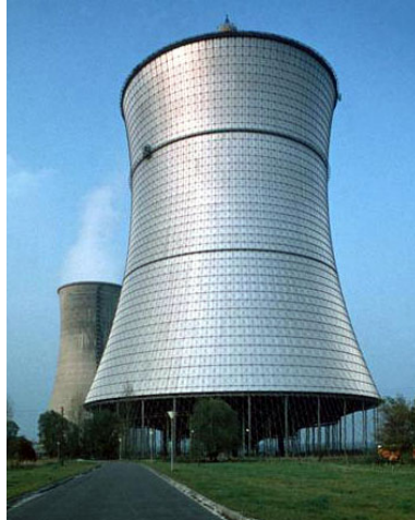
Figure 6. Dry cooling tower in foreground, wet cooling tower in background in the THTR-300 pebble bed Th reactor, Germany.
