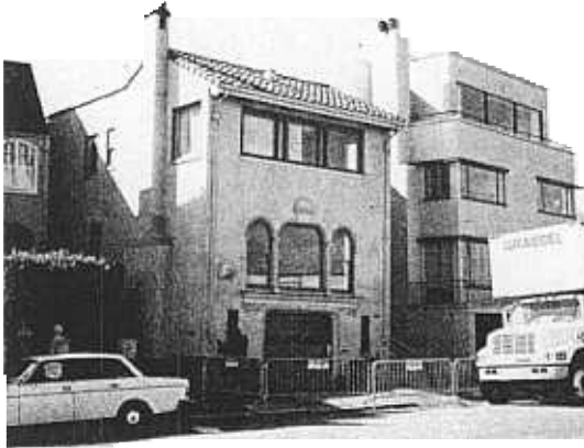
Figure 3.3 Settlement and tilting of buildings in the Marina District of San Francisco
