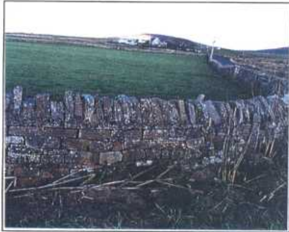
Localised drystone walls around large farms and on unstable sand landscapes. Occasional stone slab fence.
