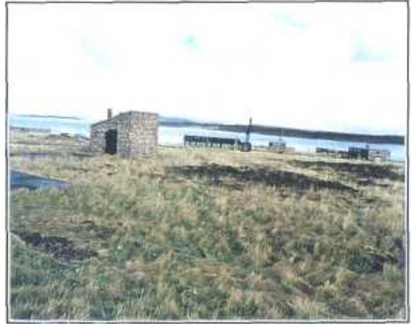
Derelict Military Structures of World War II.
