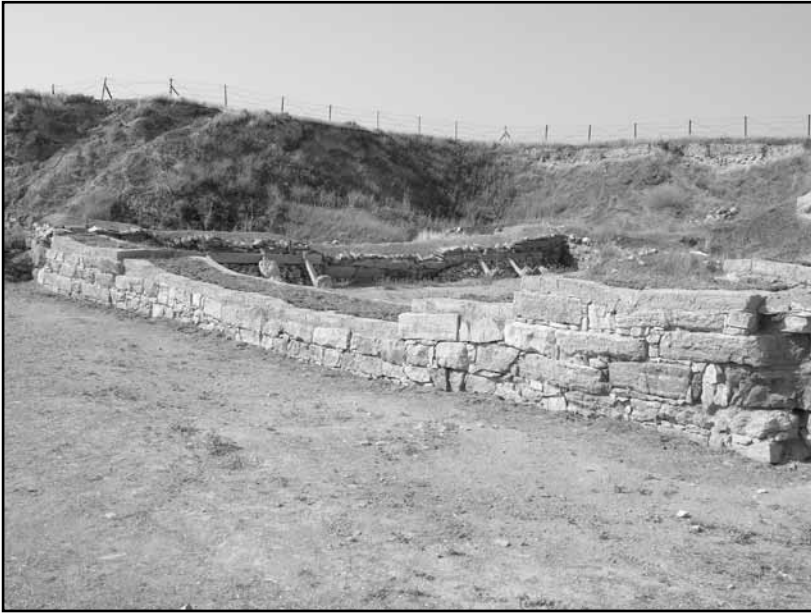
Fig. 8: Terrace Building 2, northeastern wall, after completion of repairs and soft capping.
