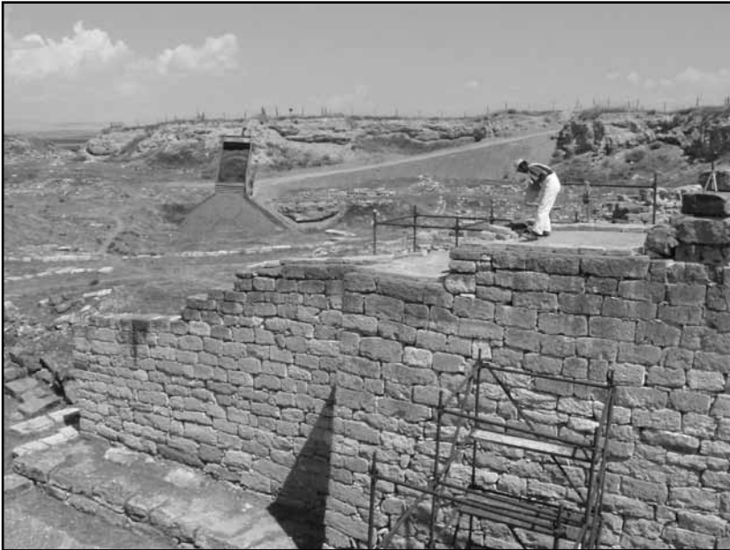
Fig. 11: Citadel Gateway, southern wall of north court, during capping process.
