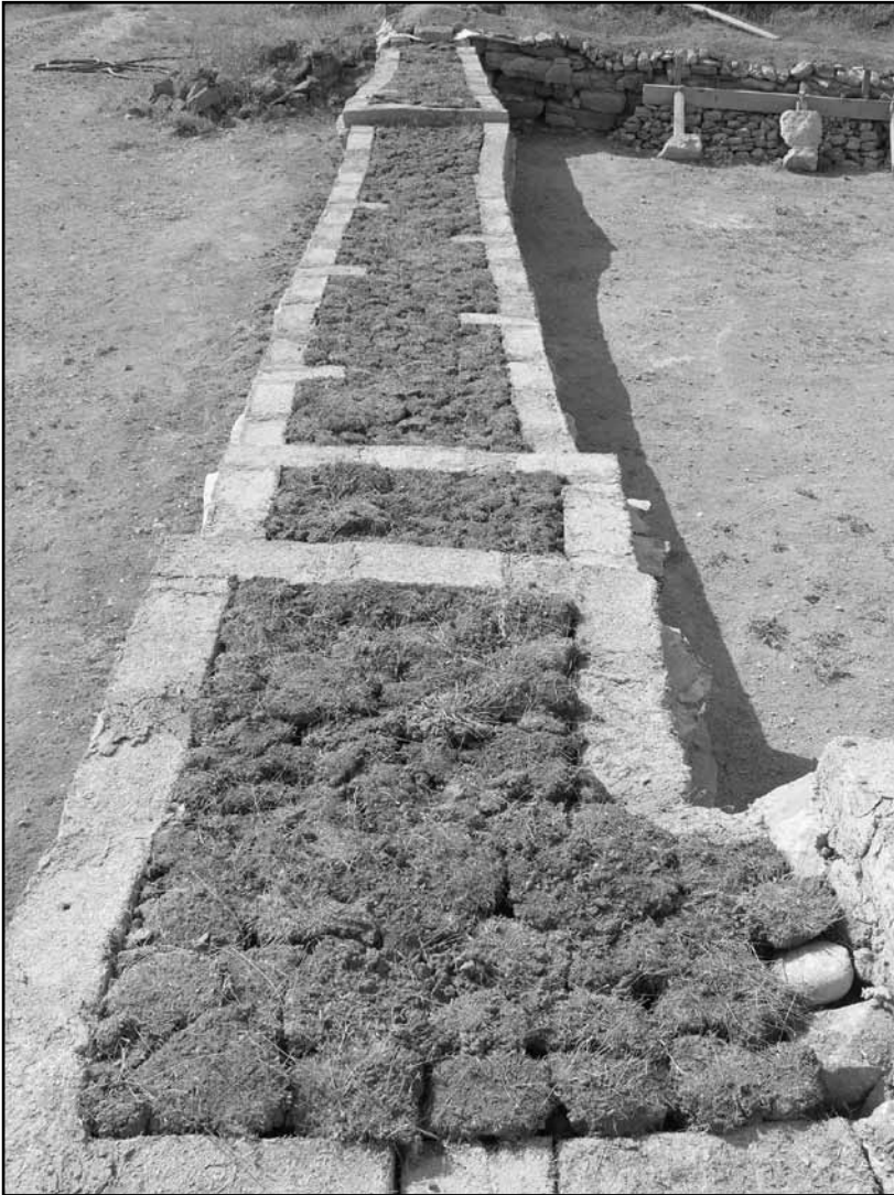
Fig. 7: Terrace Building 2, northeastern wall, after completion of soft capping.
