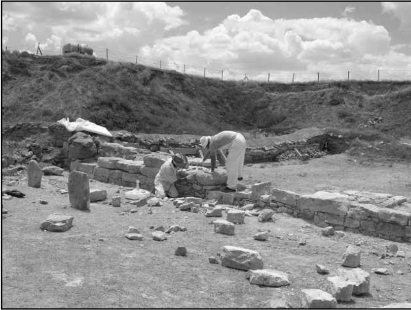
Fig. 5: Terrace Building 2, northeastern wall, during repairs and stone replacement.
