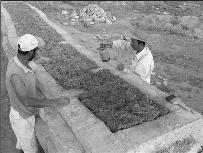
Fig. 6: Terrace Building 2, northwestern wall, during installation of soft capping.
