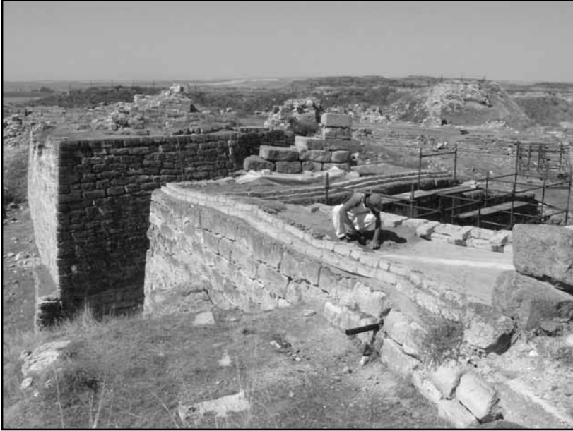
Fig. 10: Citadel Gateway, eastern wall of north court, during capping process.
