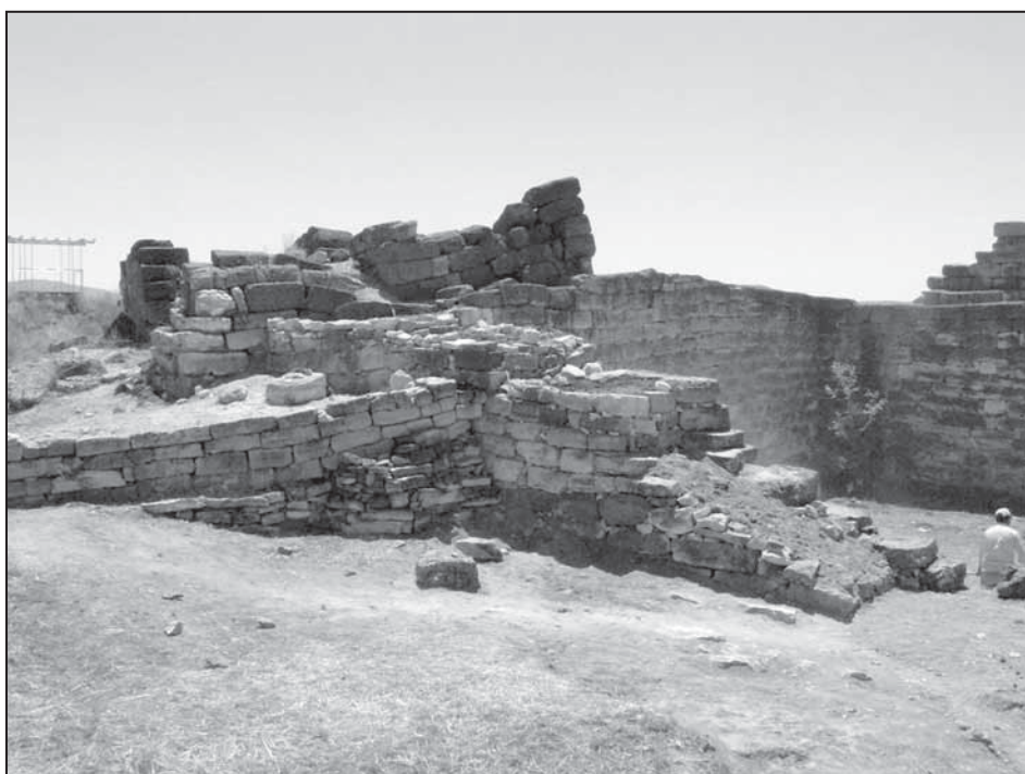
Fig. 13: North wall of Early Phrygian Citadel Gateway complex, with soft capping of vegetation concealing underlying waterproofing and drainage materials
