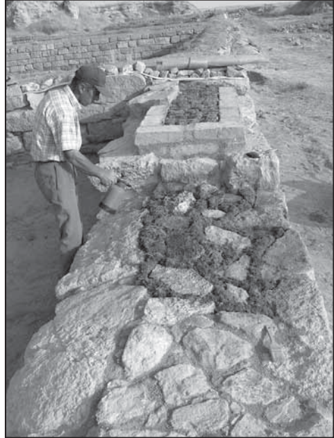
Fig. 10: Rear (northeastern) wall of Terrace Building 2, with experimental soft cappings.
