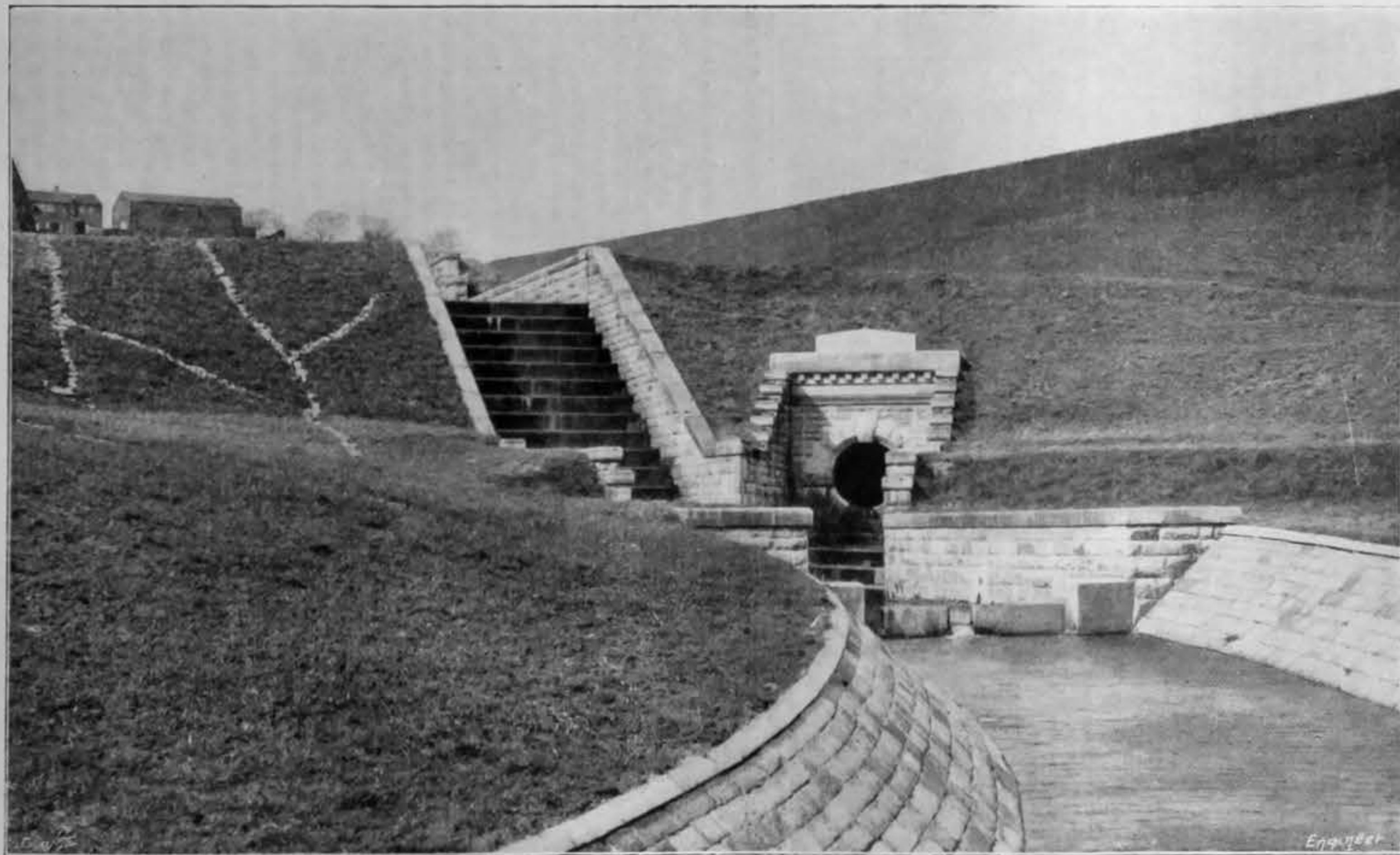
TUNNEL OUTLET, LOWER BYE-WASH, AND GAUGE BASIN
