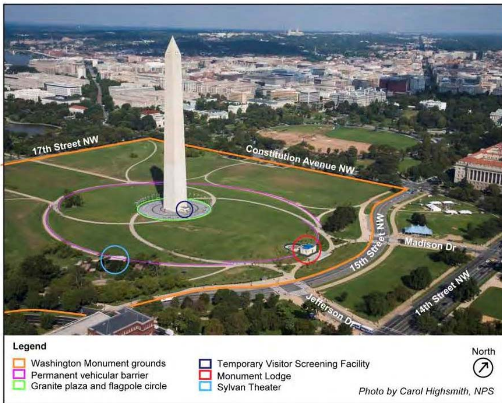
Figure 2: Aerial of project site
