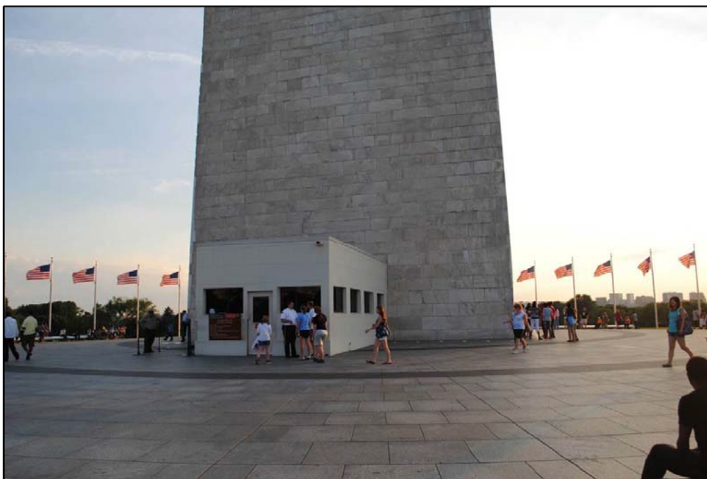
Figure 3: Existing visitor screening facility constructed in 2001
