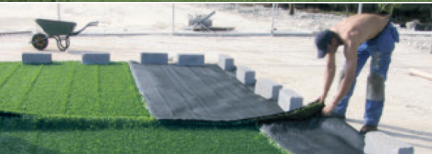
Laying an artificial pitch on the Seychelles.
