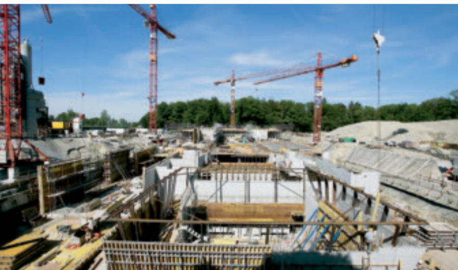
Looming large: the new Home of FIFA is taking shape.
