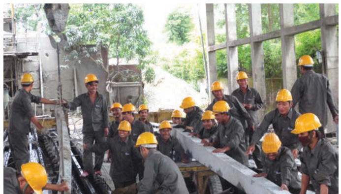
Amlekhgunj Concrete Pole Plant
