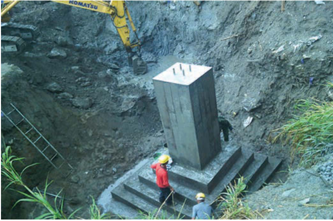
Bhulbhule –Middle Marsyangdi Transmission Line Tower Foundation Work
