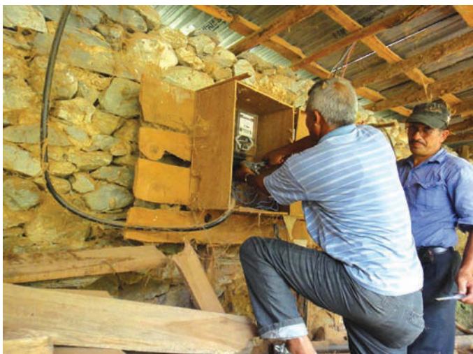
Meter resealing being done by NEA Employee
