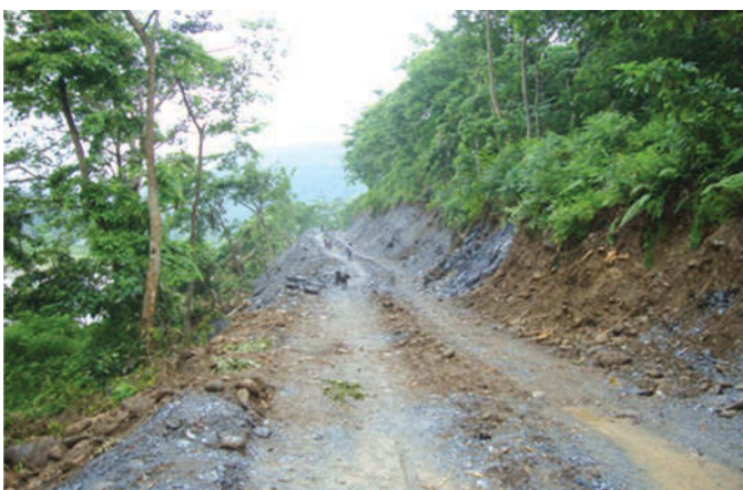
Under construction access road to Powerhouse site.
