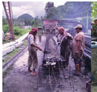
PSC Pole Production at Kotre Pole Plant
