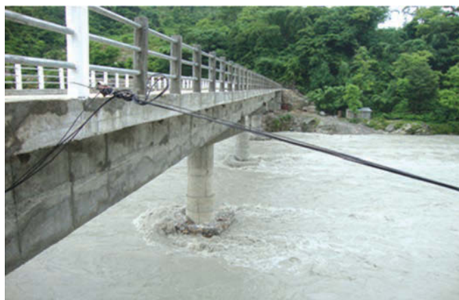
RCC Bridge over Seti River
