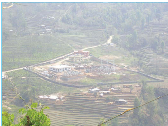
Godak (Ilam) 132/33 kV substation
