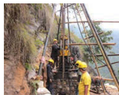
Core drilling at Tanahu HEP
