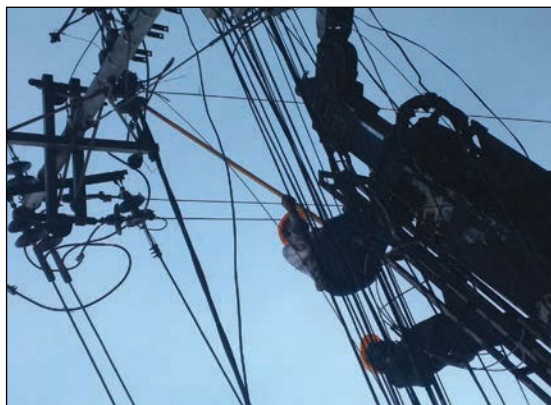
NEA Staff at work for services restoration after April, 2015 Earthquake
