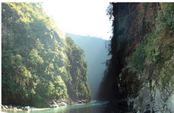
Proposed Dam site of Tanahu Hydropower Project
