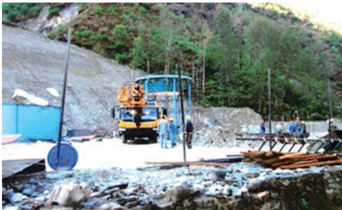
Batching Plant at Headworks
