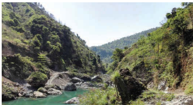
Andhikhola Dam Site
