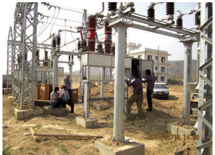
Construction Works of 33 kV S/S
