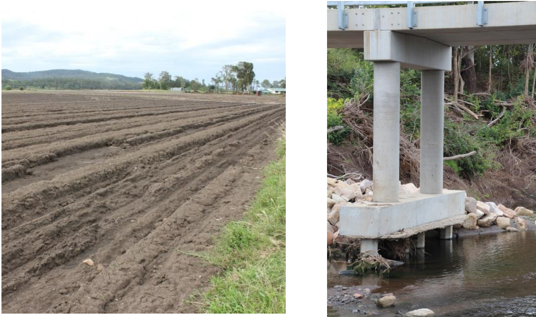
Figure 2: Damage sustained in the January 2013 flood of Laidley Valley (a) erosion of agricultural fields down to the controlled traffic line and, (b) undermining the foundations of bridge infrastructure caused by deepening of the Laidley Creek.
