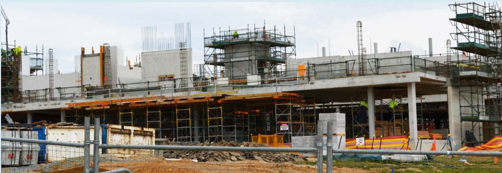
The new forensic facility under development
