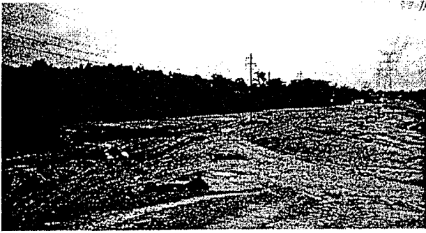
Plate 3 Floodway under Construction on Southern Bank of Toongabbie Ck
