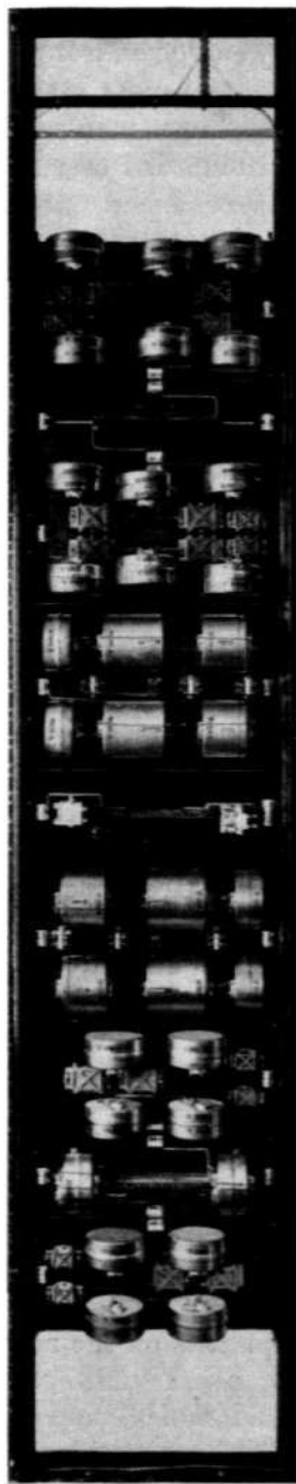
R 1452 Fig. 12. Line Filter Bay (rear view).
