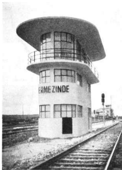
Fig. 1 Interlocking cabin at Ermezinde
