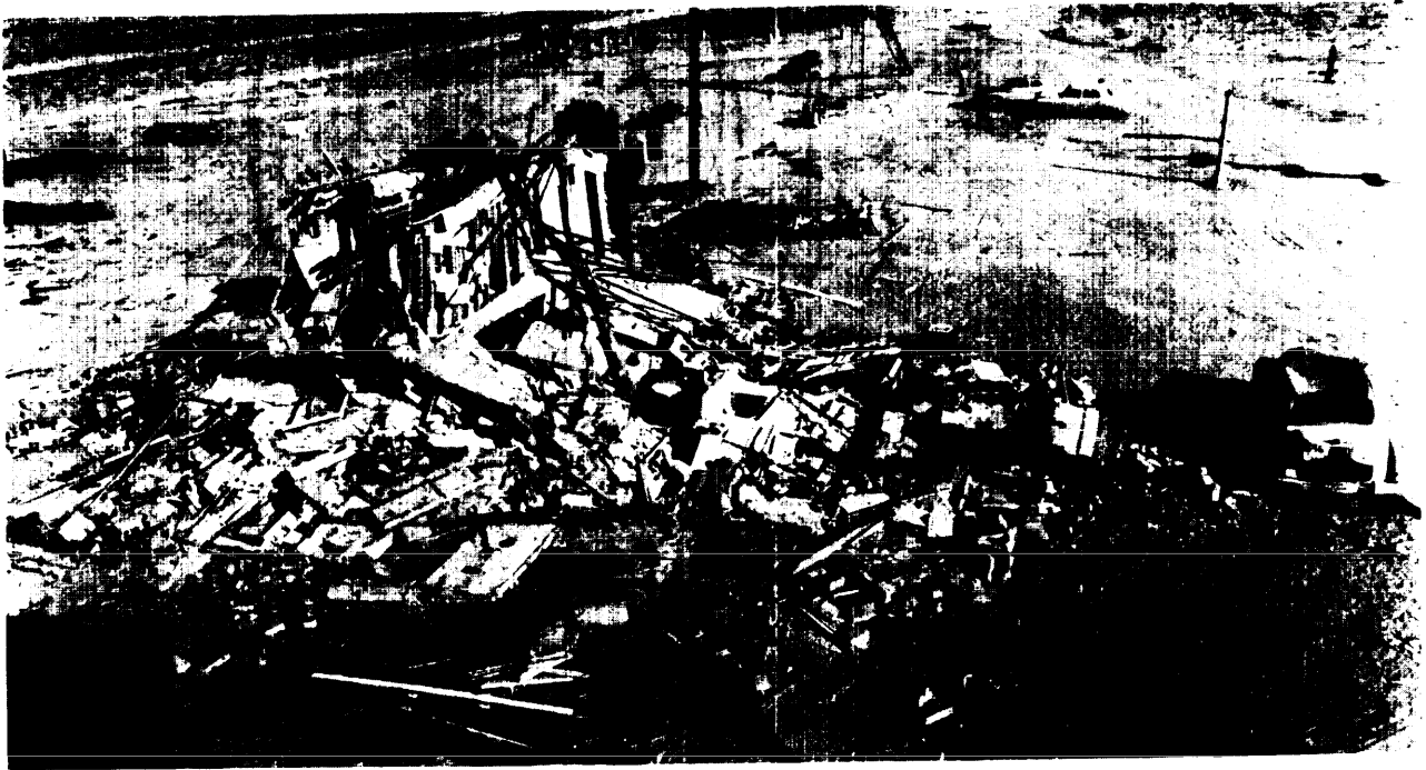
Damage to unreinforced brick house (5-psi overpressure)
