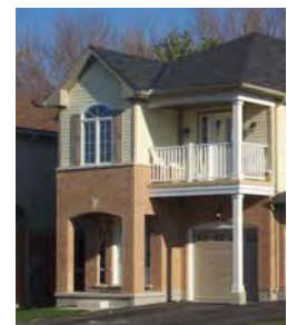
Putting a habitable storey atop the garage
