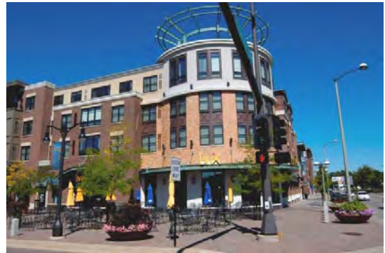
Well integrated corner building and plaza can serve as a landmark to enhance the cognition of the node or gateway
