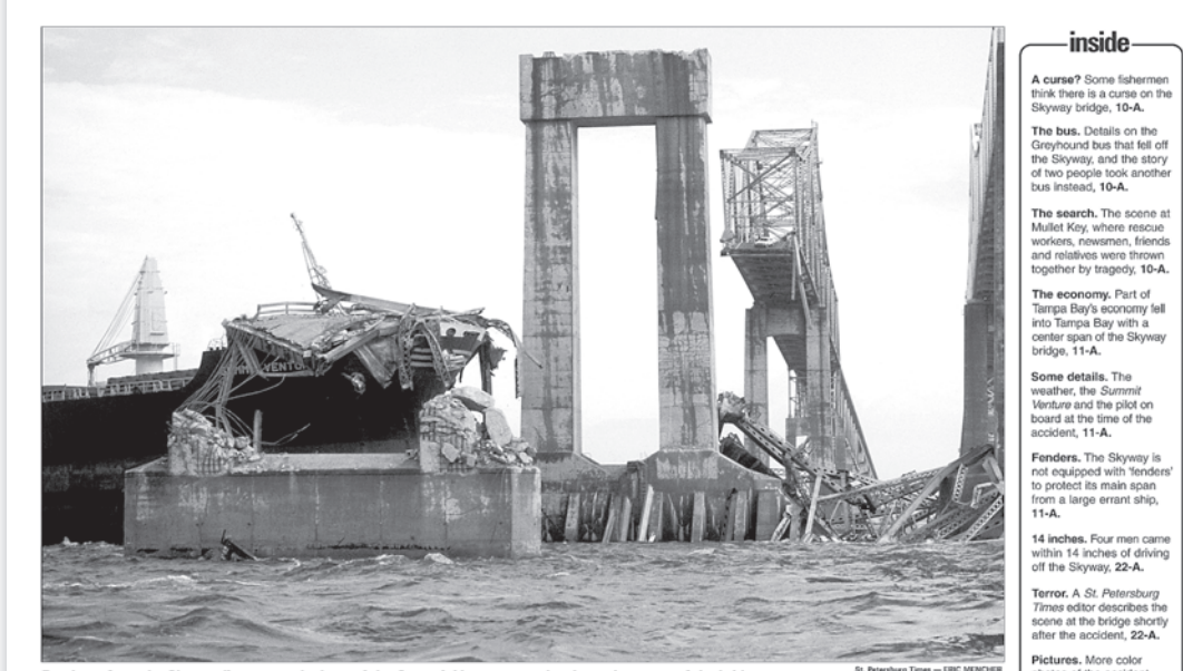
Roadway from the Skyway lies across the bow of the Summit Venture near the sheared support of the bridge
