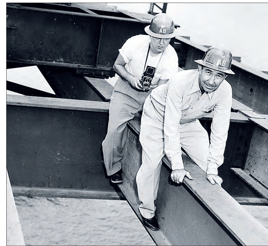
When they reached the still-incomplete middle span of the original Sunshine Skyway, outdoors writer Rube Allyn, front, and photographer Bob Moreland gingerly inched their way across.
