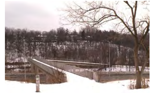
Footbridge at St. Paul Crescent
