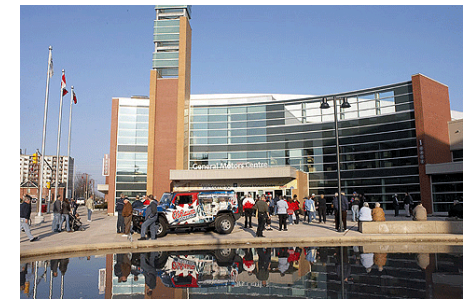
Recently completed General Motors Centre, Oshawa
