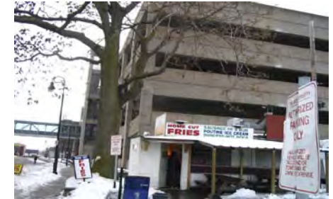
View of the existing Carlisle Street Garage
