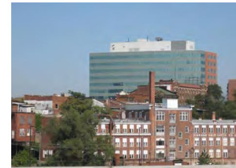
Both MTO Building and the Canada Hair Cloth building have significant Downtown presence
