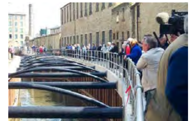
Canal Restoration in Huddersfield, England.
