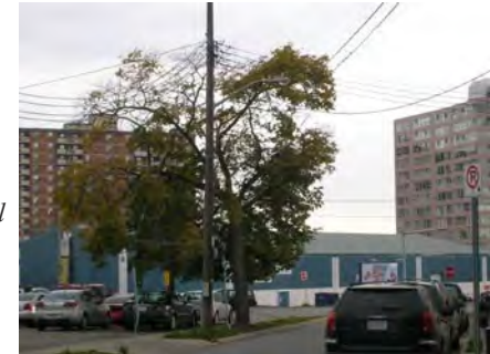
View of Arena from St. Paul Street
