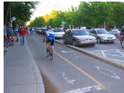
A two-way, physically separated bike lane on a busy avenue, Montreal
