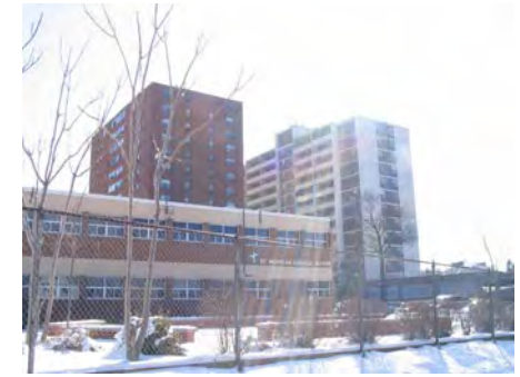
View of apartment building and school property, between North and Church Streets
