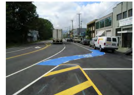
New clearly marked on-road cycling lanes, Vancouver
