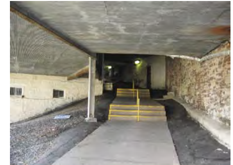
Existing stair connecting St. Paul Street and Lower Level Parking Lot
