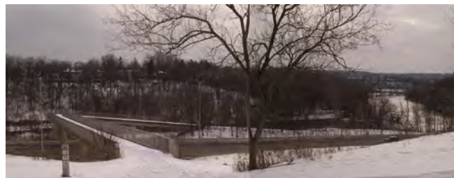
View of the pedestrian bridge into Twelve Mile Creek Valley
