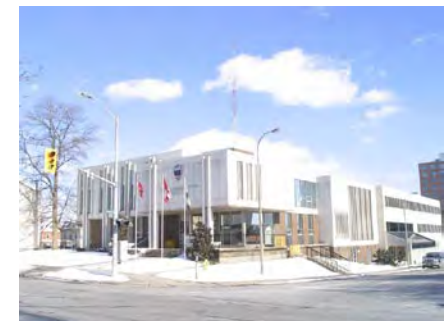
Niagara Regional Police Headquarters, Carlisle and Church Streets
