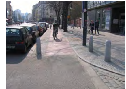
Bike lanes can share sidewalk space but should be clearly separated from pedestrians, Berlin
