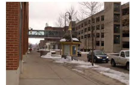
View of Carlisle Street Parking Garage
