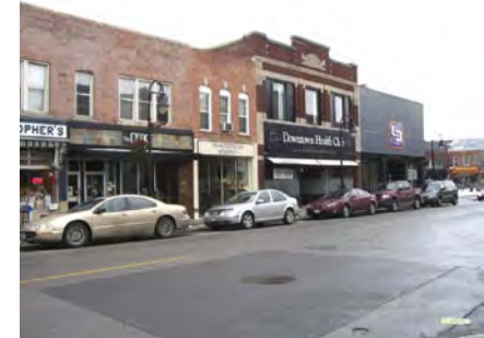
James Street, looking south east, towards St. Paul Street
