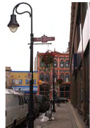
Access to May Alley, which function as an east-west service alley parallel to St. Paul Street
