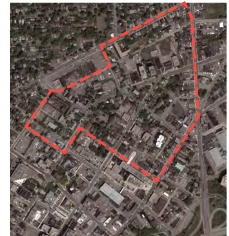
Aerial view of area
