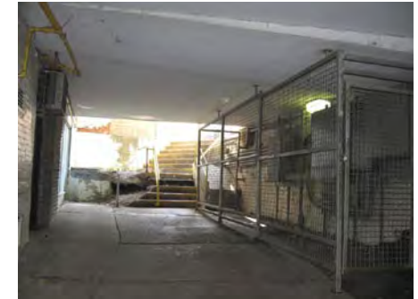
Existing stair access up to St. Paul Street
