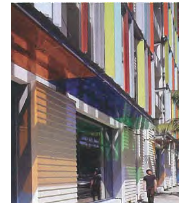
Example of a new mixed-use development, Santa Monica Civic Centre Parking Garage Complex
