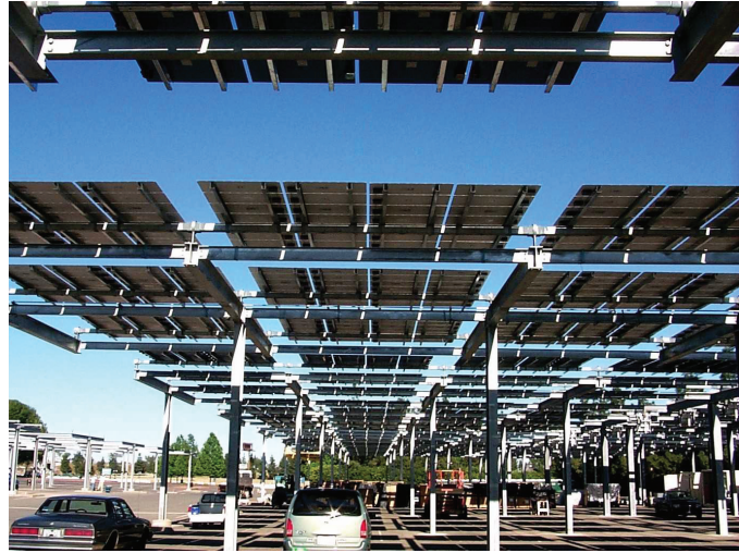
This PV system at the Cal Expo in Sacramento, California, was installed in September 2000. The 540-kilowatt PV system produces enough energy to power about 180 homes. The solar arrays serve as a shaded oasis for 1,000 cars in a desert of scorching blacktop. (Photo Credit: Kyocera Solar)
