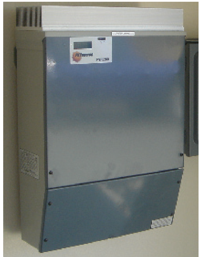
Inverters come in a wide range of styles, classifications, and optional features. The one shown here is manufactured by PV Power and includes a digital read out. (Photo Credit: Rodney Slaughter)
