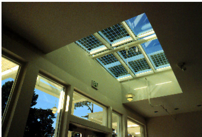
Laminated to the skylight glass are photovoltaic cells that produce electricity as well as serve as an element in the shading and day lighting design at the Thoreau Center for Sustainability, Presidio National Park, San Francisco, California. (Photo Credit: Lawrence Berkeley Lab)
