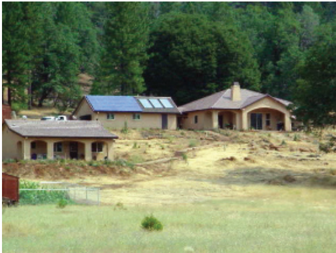
This rural home in northern California uses both an off-grid PV system along with a solar thermal system. (Photo Credit: Alan Wing)
