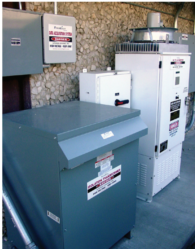
The inverter for this system is significantly larger than those you would expect to find on a residential system. (Photo Credit: U.S. Postal Service)
