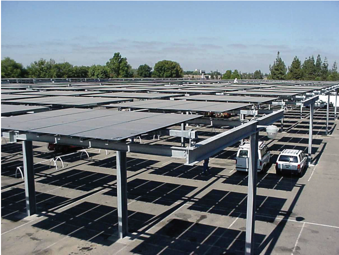
This PV system at the Cal Expo in Sacramento, California, was installed in September 2000. The 540-kilowatt PV system produces enough energy to power about 180 homes. The solar arrays serve as a shaded oasis for 1,000 cars in a desert of scorching blacktop. (Photo Credit: Kyocera Solar)
