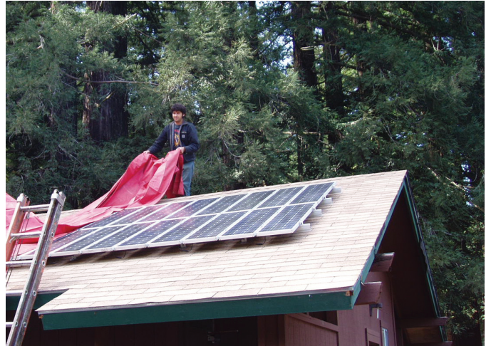
A fire department salvage cover was employed in California only to discover that while it significantly reduced the Sun’s intensity and the electrical energy that it generates—it did not completely block out the Sun and the system still generated enough volts and amps to shock a potential victim. (Photo Credit: Marc Fontana)
