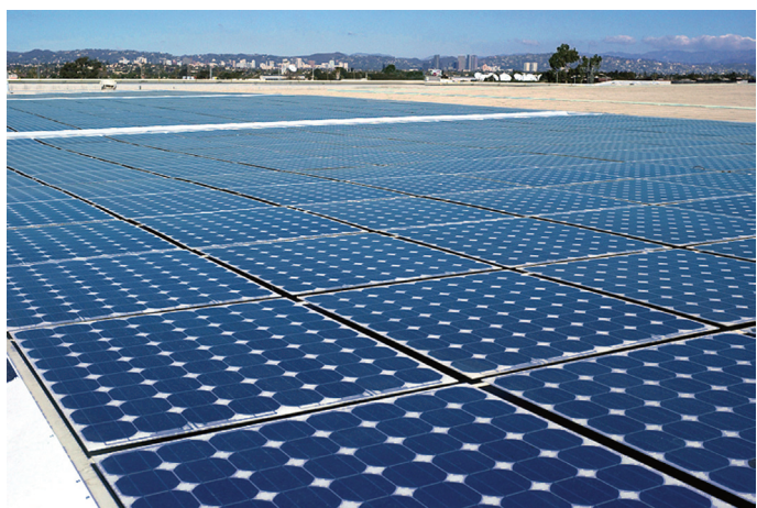
The roof top of the USPS processing and distribution center in Marina Del Rey, California shows the use of a 127 kw monocrystalline PV system. (Photo Credit Power Light Corporation)
