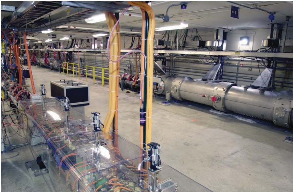
Figure F-1. Photograph of an FEL Facility
