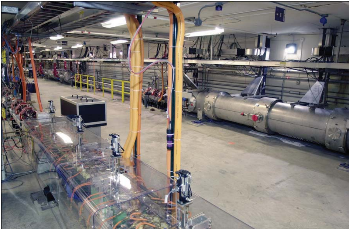
Figure F-1. Photograph of an FEL Facility
