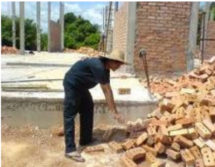
3D work situation
