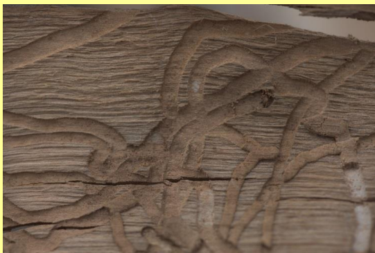
Wood-boring larval damage to a eucalypt trunk
