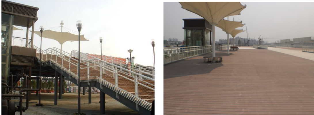
Figure 3-10: Sun-Shading System on Elevated Pedestrians' Walk
