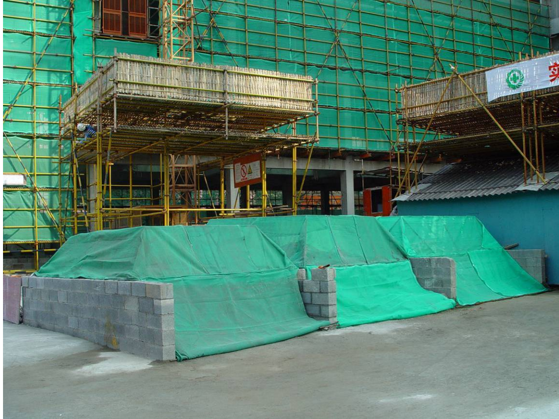
Figure 2-20:Fugitive Dust Pollution Control on Construction Site
