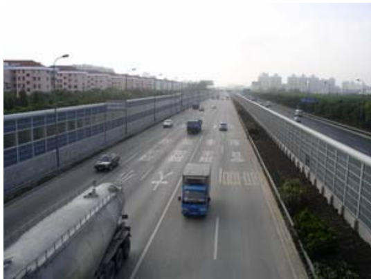
Figure 2-26: Noise Barriers in Outer Ring Road
