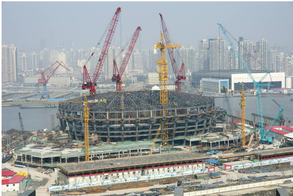
Figure 3-26: Photo of Performance Center under Construction (by Xu Zhengkui)
