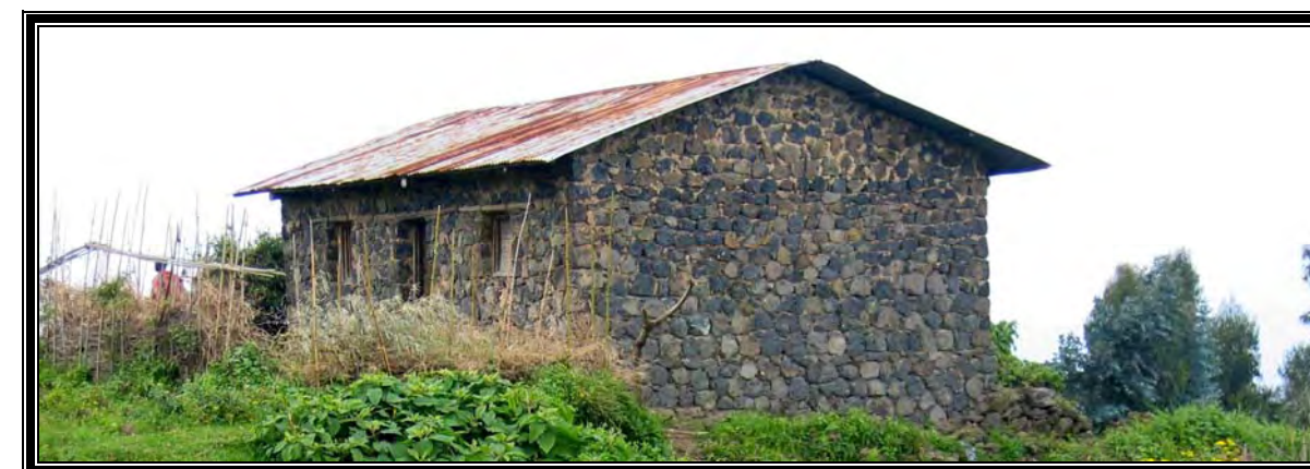
Rwandan houses at the edge of PNV use a lot of lava rocks.
