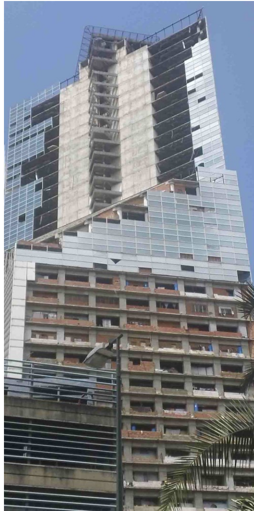
Fig. 2 Exterior view of the “Torre de David” in Caracas.
