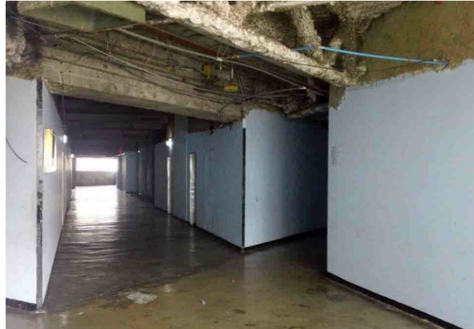
Fig. 6 Interior corridors of Torre David
