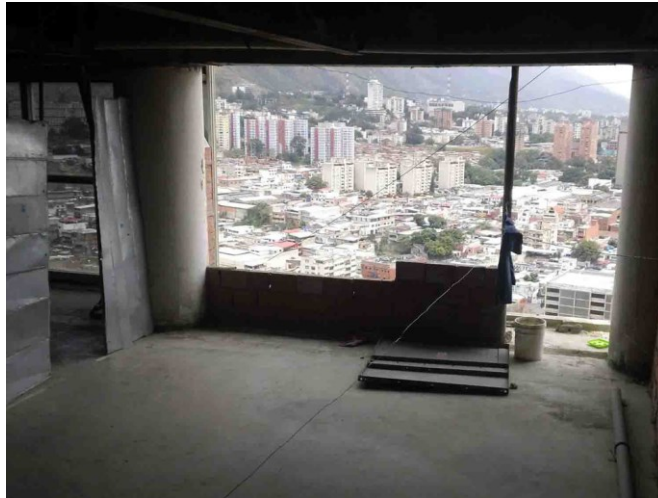
Fig. 10. Interior of a non-improved dwelling with a complete open fenestration.
