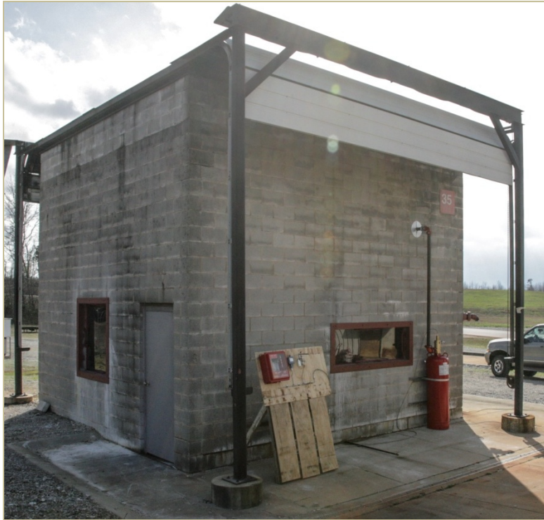
Figure 2: Fire test enclosure
