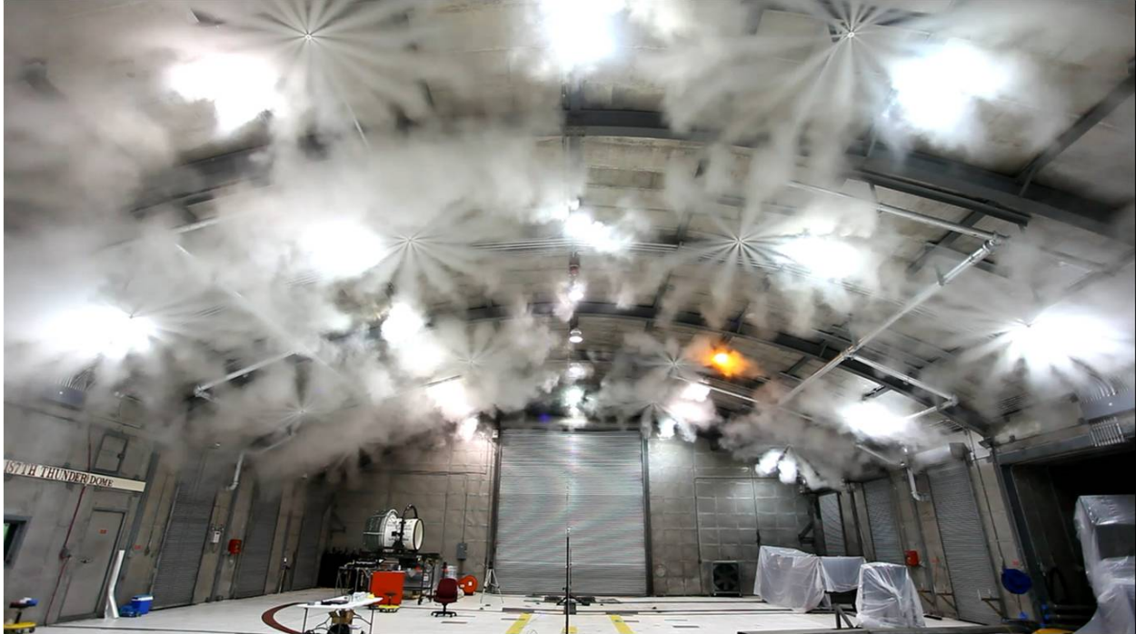
Fig 8: U.S.A.F. AF37T-10 hush house Full-scale Agent Concentration Test
