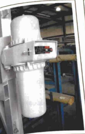
Exhibit 501.15 An explosion-proof enclosure for a motor control and circuit breaker. (Courtesy of Appleton Electric Co., EGS Electrical Group)
