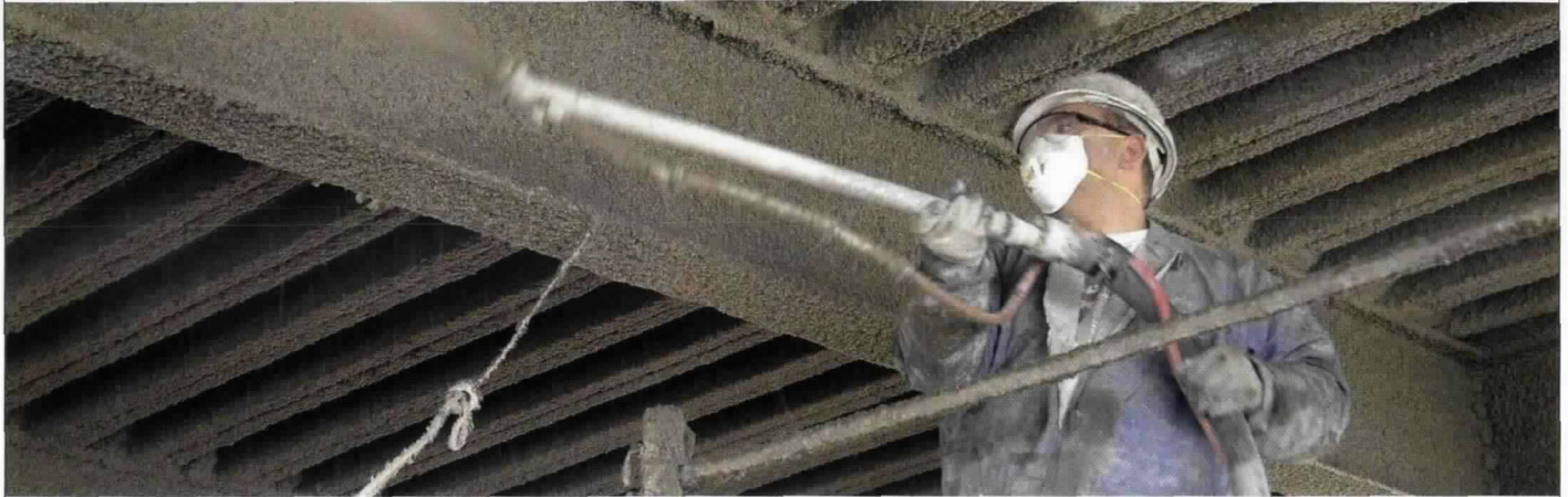
A construction worker sprays fireproofing inside 7 WTC.
