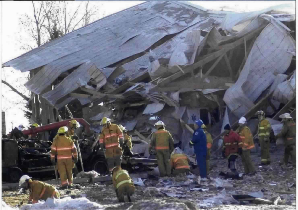
Firefighters and state inspectors search through the remains of a fire hall destroyed by an explosion.
