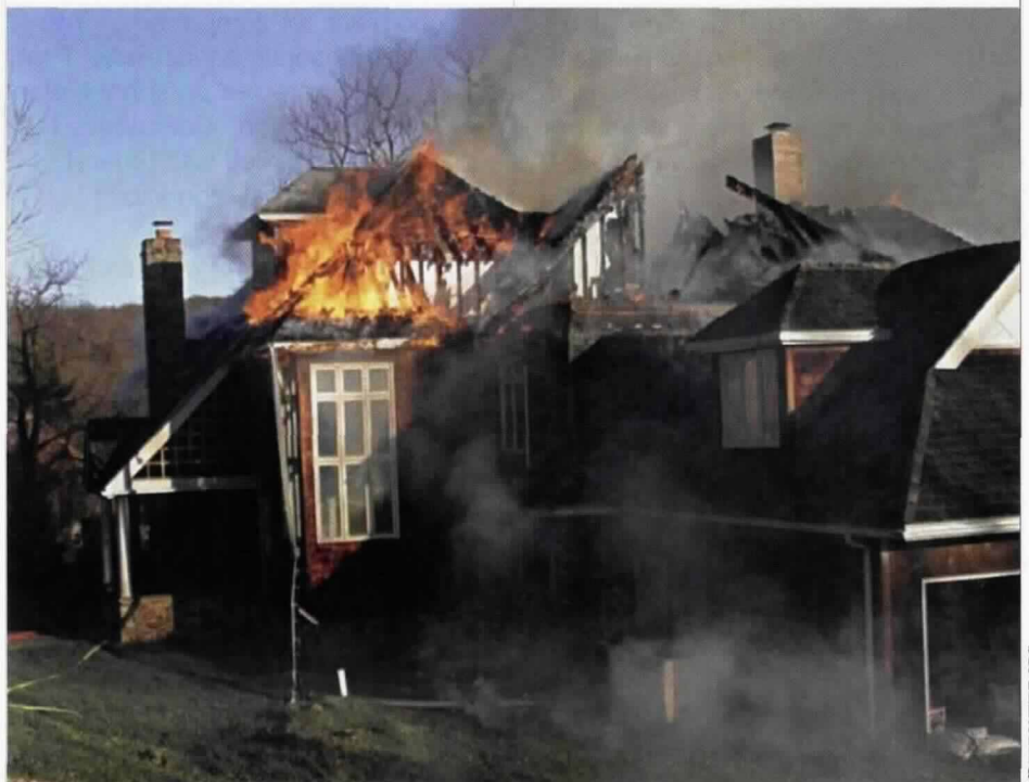
A passing motorist saw smoke coming from the roof of this three-story Pennsylvania house and alerted the fire department. The wood-frame home's fire detection system had been disabled.
