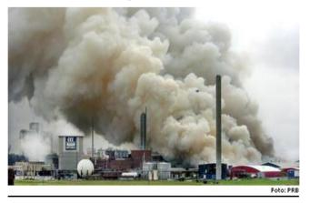
Figure 1 : visible smoke threat from ternary type NPK decomposition (Sweden, July 2004)
