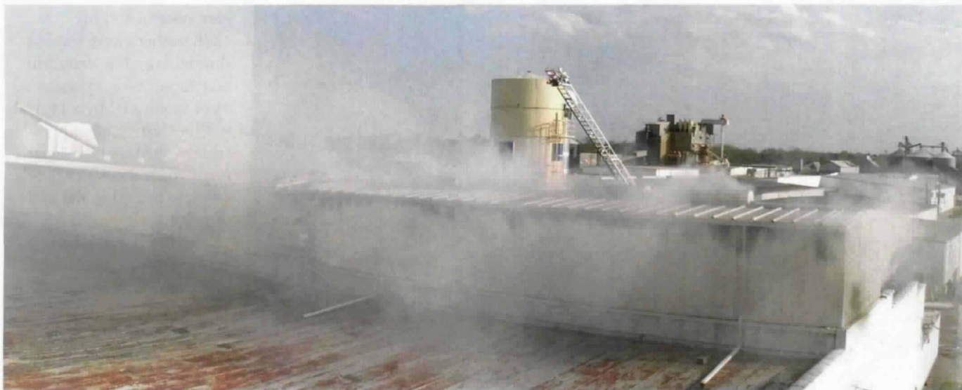
Excessive heat from a worn bearing or fan belt motor is, according to investigators, the most likely cause of this processing plant fire.
