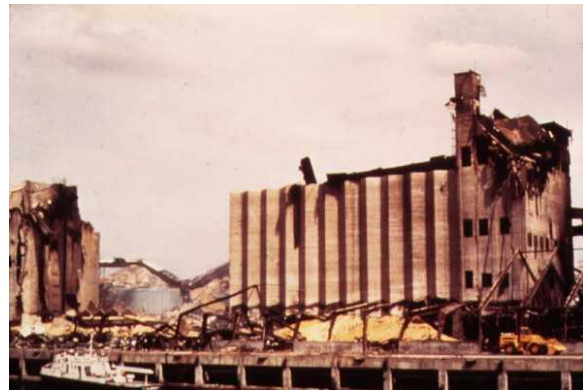
Figure 2 - Houston, TX Explosion 2/76
