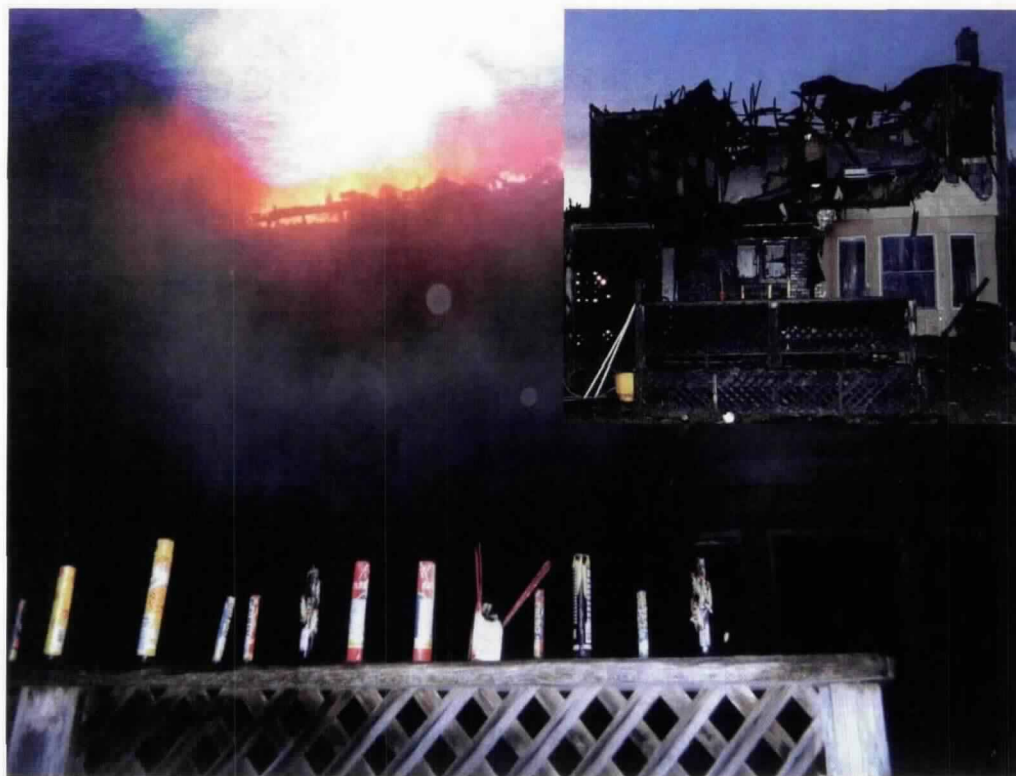
Independence Day fireworks was responsible for this fire on the back deck of a single-family home in Michigan. The house (inset) was heavily damaged, but no one was injured.
