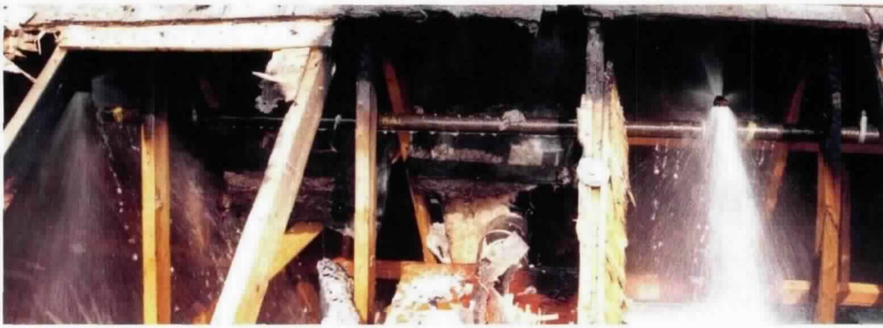
Sprinklers controlled this fire, started by a carelessly discarded cigarette, as it spread up the exterior siding of a nursing facility.
