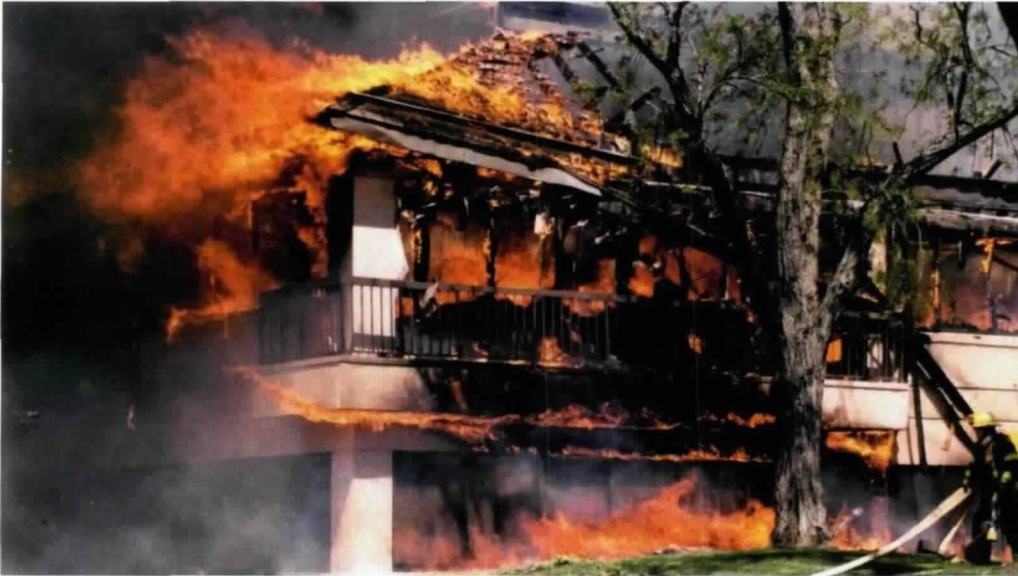
An office building in Pennsylvania burns on May 7, 2001. The electrical fire broke out in a void space above the ceiling area of the second floor. A full collapse of the roof occurred within minutes of the firefighters arrival. One firefighter was injured. Loss to the structure was $4,000,000.
