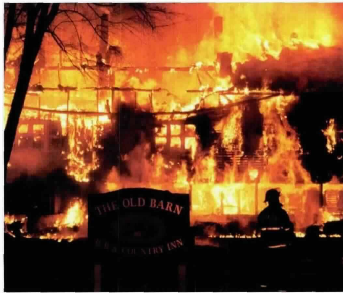
Heat and flames escaping from a flue or firebox ignited concealed structural framing of this bed and breakfast.
