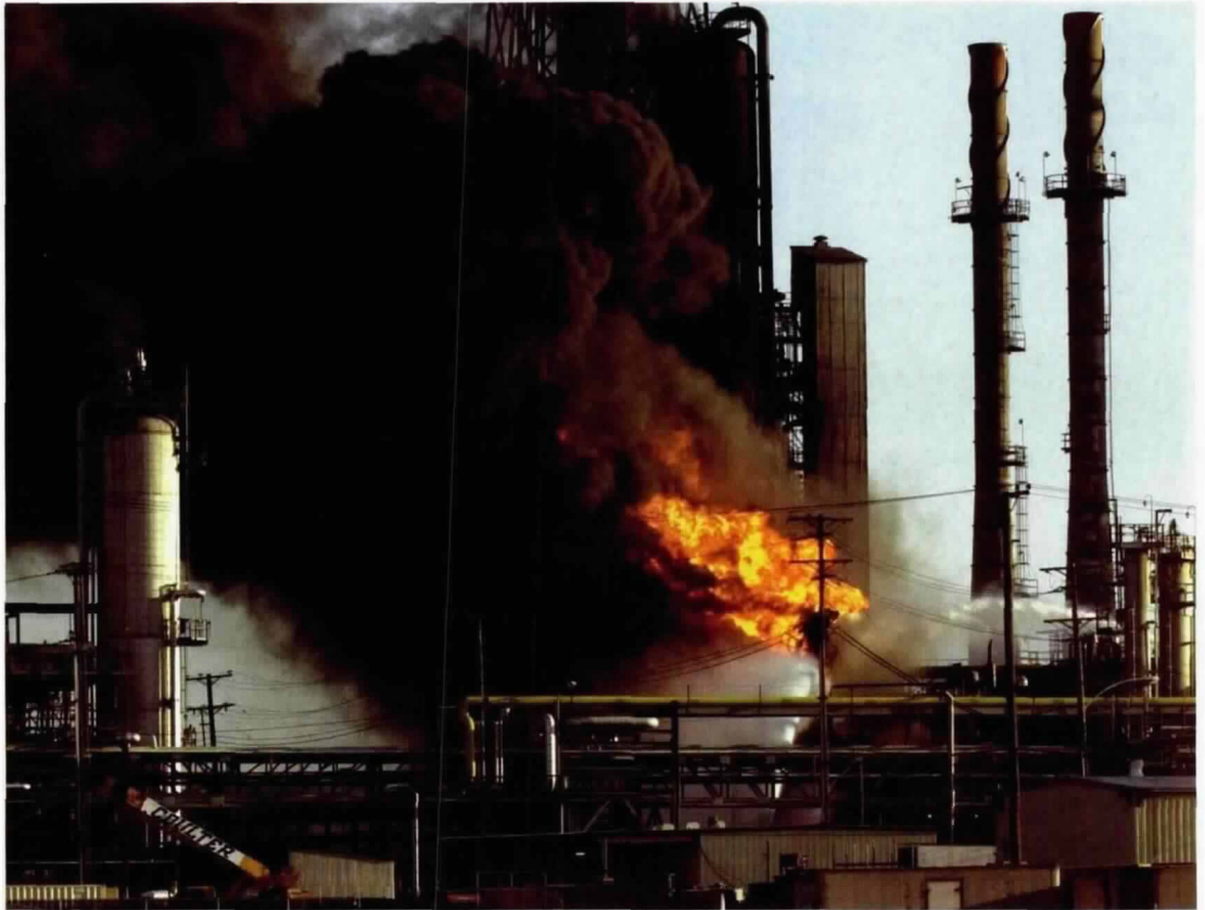
A blaze burns at a California refinery on April 23, 2001. The fire shot huge balls of fire dozens of feet into the air and sent plumes of black smoke billowing over the area, but no one was injured and no evacuations were ordered.
