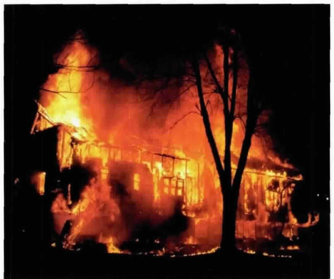
This unsprinklered bed and breakfast was destroyed in a $1.4 million fire that spread undetected in concealed spaces for hours.
