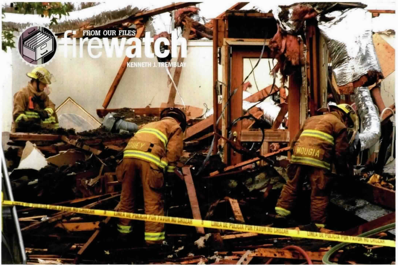
Natural gas leaking under the floor of this single-story house exploded, killing two people and injuring five others.
